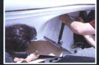
TEP 9: Drill the two holes, countersink each to prevent chipping, apply the adhesive sealant tape, dab the sheet-metal screws with sealant and mount the transom bracket.
